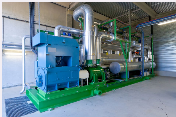
Module ORC 550 kWe - SERM, Montpellier
